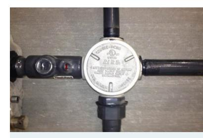
This PVC Coated Conduit was installed with an uncoated GUA fitting, which could compromise the performance of the installation. When installing PVC Coated Conduit it is important to create a sealed system. Knowledge of PVC-Coated Conduit regulations and proper installation is essential for success of a project. Graduation from Corrosion College ensures your project will succeed in a corrosive environment.
